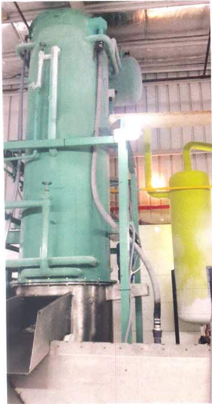
TUBE ICE EVAPORATOR (AMMONIA)
